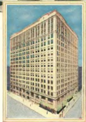
The new Adams-Franklin Building, Chicago —above is view of rubber flooring in elevator lobby
